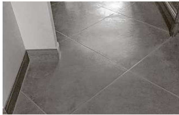
This concrete floor is stained to look like large squares of Saltillo tile. Melanie Bowles of A Creative Design did treatment on the concrete floor.
