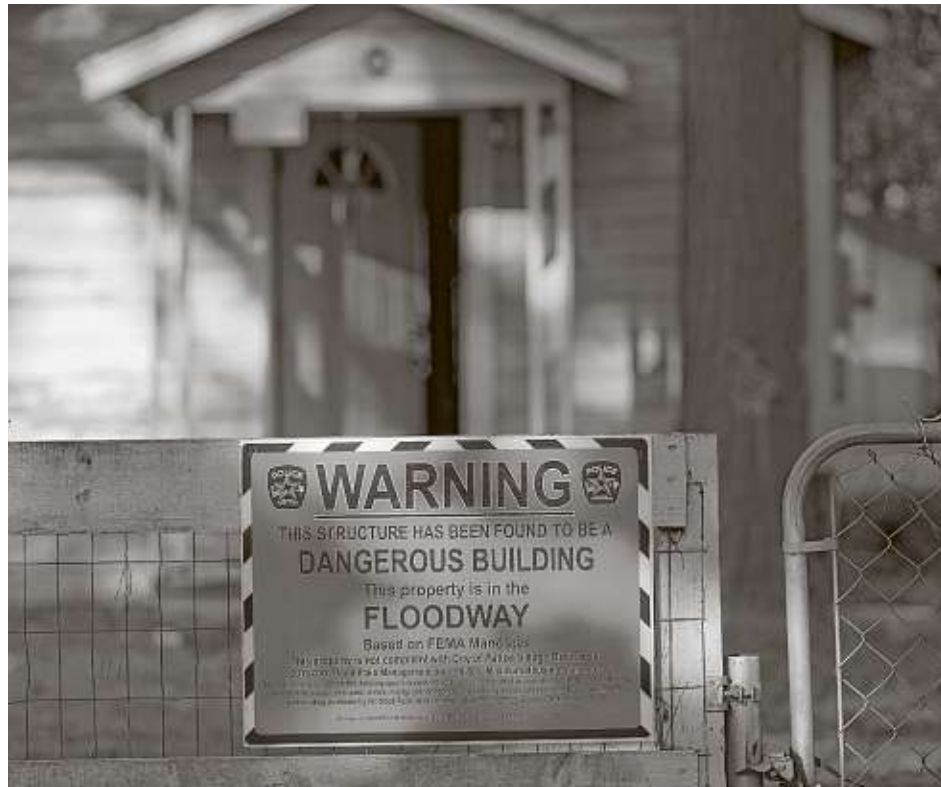
A FEMA warning sign is shown near a home damaged by floodwaters in Patton Village. More than 700,000 people have applied for assistance so far.
