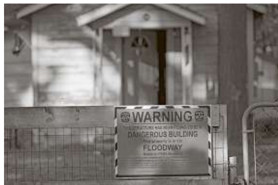
A FEMA warning sign is shown near a home damaged by floodwaters from Harvey.
