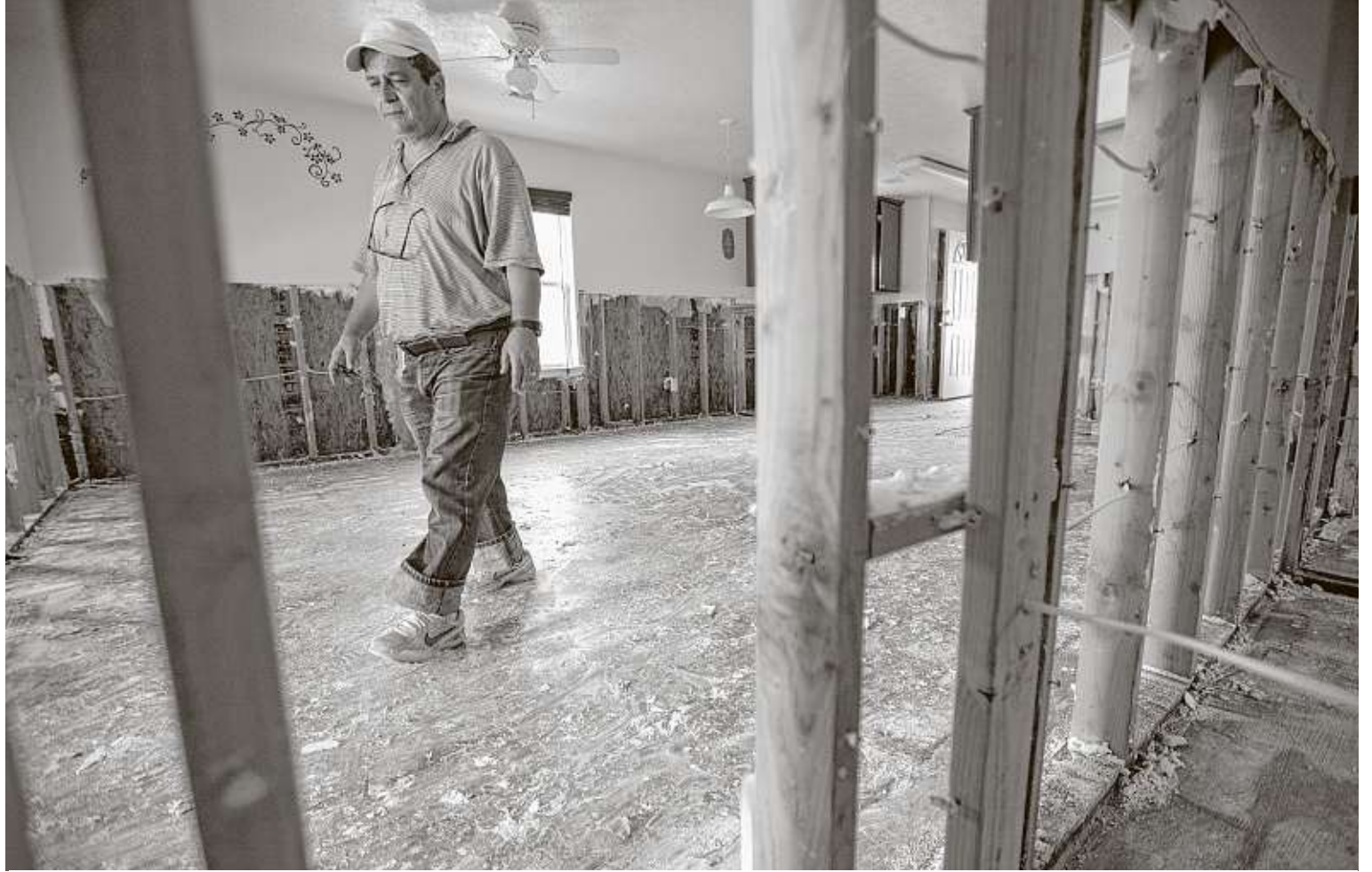
Driss Lassile walks through his house after volunteers from Habitat for Humanity helped remove drywall and carpet.
